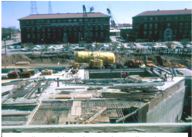
Installation of the tandem Van de Graaff accelerator under the Engineering Mall in 1968
