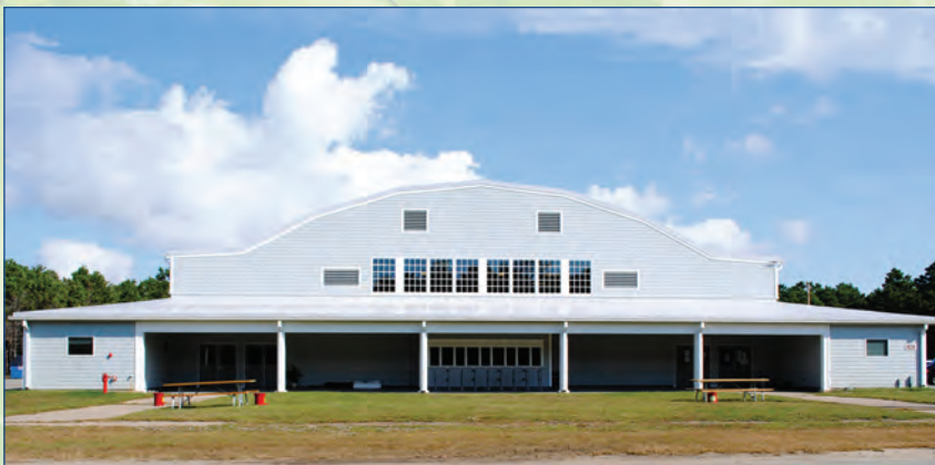
The recently-renovated Camp Edwards gymnasium.
