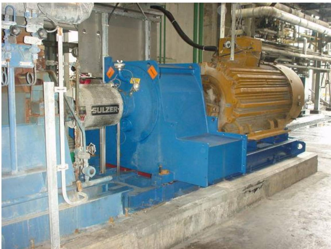
Attachment 1: Fluid Couplings in a Steam Turbine Power Plant
