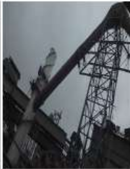
Recirculation duct tapping from Stack
