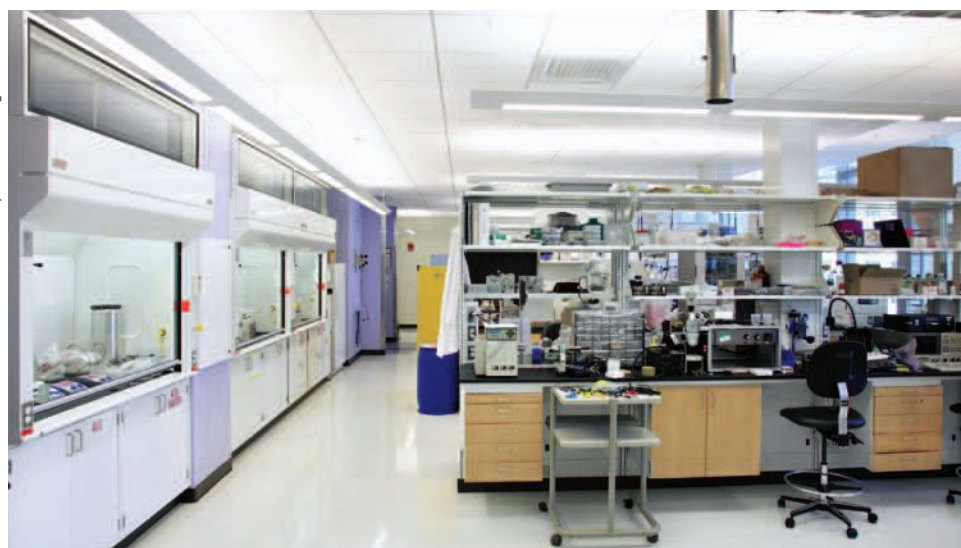
The high-performance laboratory fume hoods used in the Koch building—shown above—have an improved aerodynamic design so a lower volume of air can be passed through and still provide the same or better level of protection to the user. Energy savings accrue from having to filter, move, cool or heat, and clean less air.
