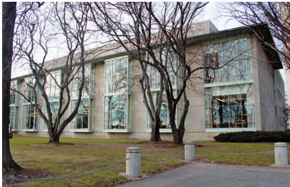
An Efficiency Forward review focusing on the operation of MIT’s Building 14 (above) led to the identification and implementation of several energy-saving changes. One finding, for example, was that fans could be run at a lower speed and still supply the correct amount of fresh air to the building.
