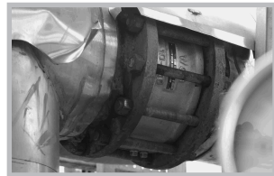
Figure 1.9 — When this non-return valve failed on a plant, hundreds of pounds a week was wasted on extra electricity for the compressor
