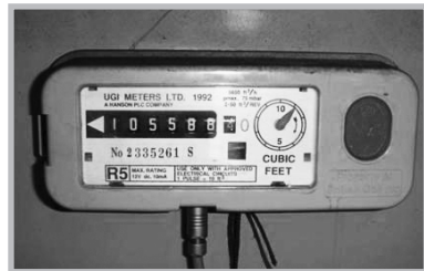
Figure 1.3 — This meter should be read as 10558840 cubic feet
