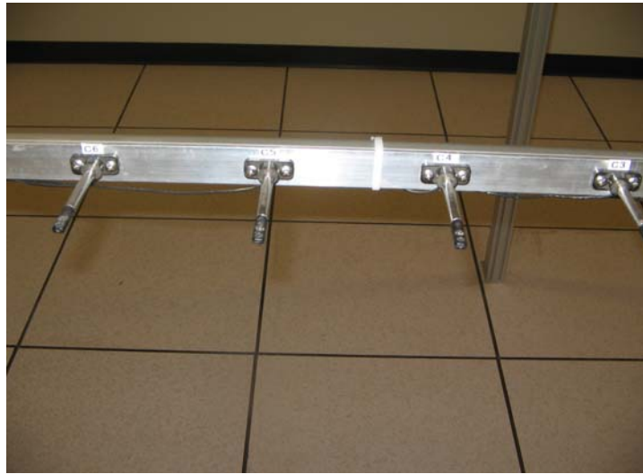
Figure 3.5 – Sensors Mounted in Testing Position
