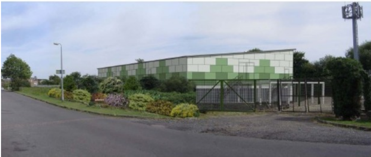
Photo Courtesy S&C Electric
