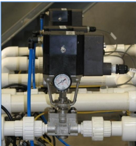
Figure 31 Control Valves FV03 and FV04 installed in the UWS.
