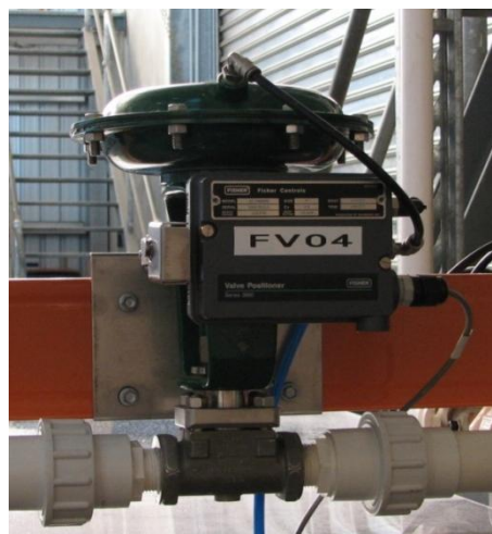
Figure 31 Control Valves FV03 and FV04 installed in the UWS.
