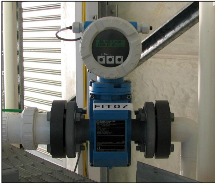
Figure 25 Promag W Magnetic Flow Meter FIT07
