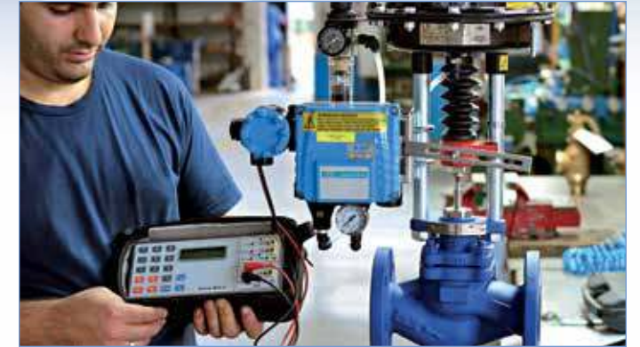
Control valve automation
