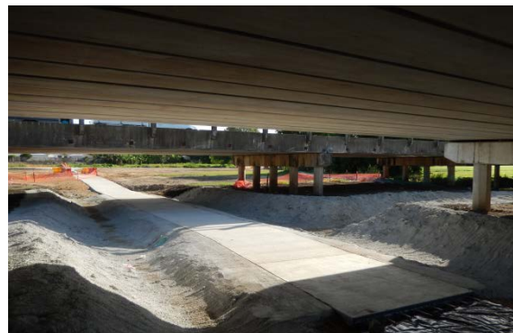
Goosepond Creek Footpath – path under existing Bruce Highway Bridges
