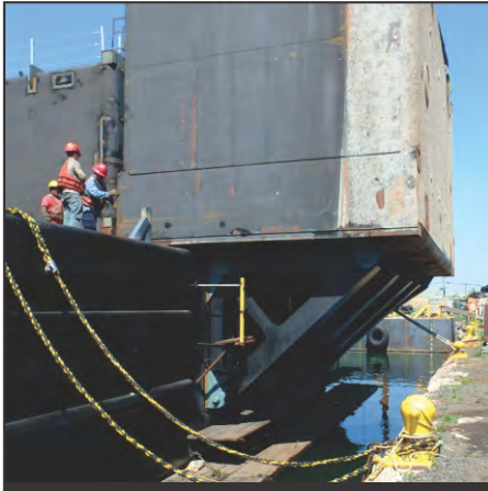
External buoyancy tank installed on to the JG BURKE
