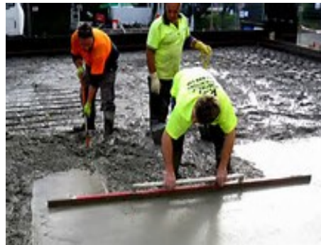
Hand-Placed Concrete
