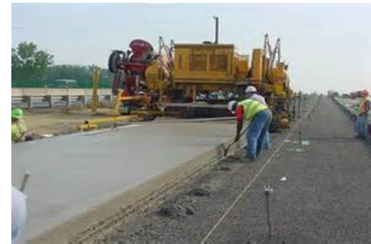
Slip-formed Concrete
