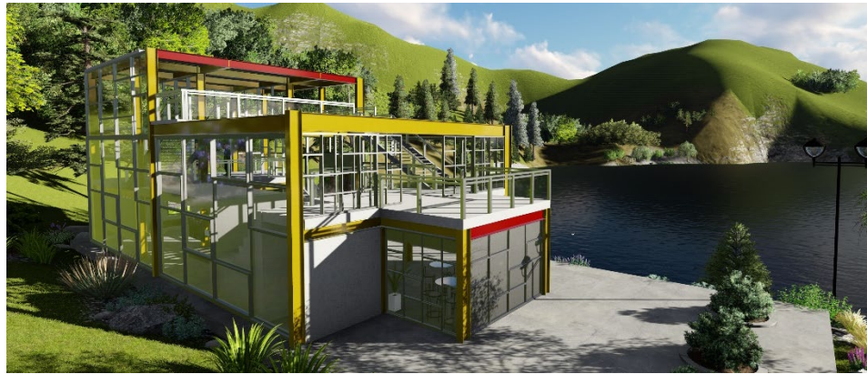
Figure 4: A steel and glass building
