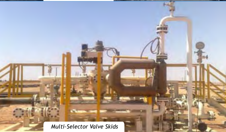
Oil Inlet Manifolds
