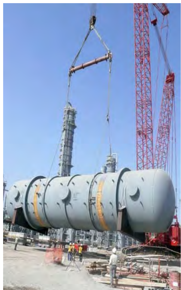
Erection of 200 ton Knockout Drum using 750 ton Crane for Sohar Aromatics Project
