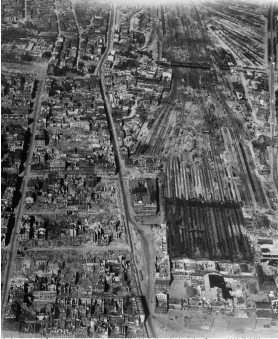
A destroyed German railway from Allied bombs during the Second World War.
