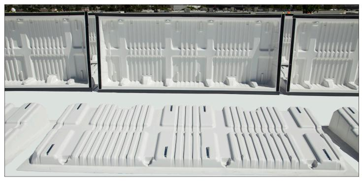
Carefully lower the ENRGY Curb unit back into position on the roofing surface and use a 10 lb (4.54 kg) weighted roller to apply pressure to the topside of the flanges.
