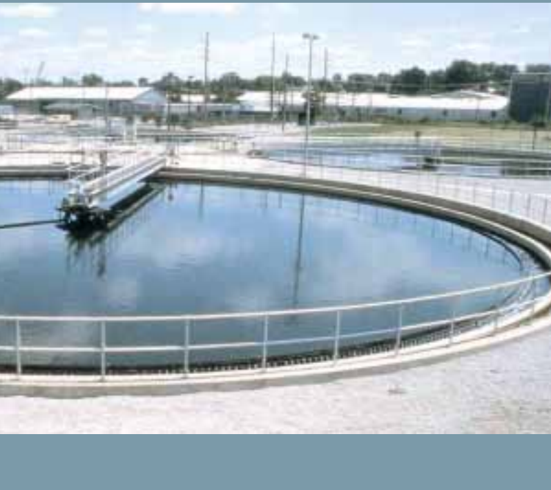
Peripheral Feed - Peripheral Take-Off Clarifier—Middle East Project was able to reduce the number of clarifier units from ten to six, providing a significant savings in capital cost.
