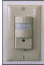
Infra-red sensor detects occupancy.
