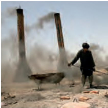
Movable Chimney Bull's Trench Kiln (MCBTK)
