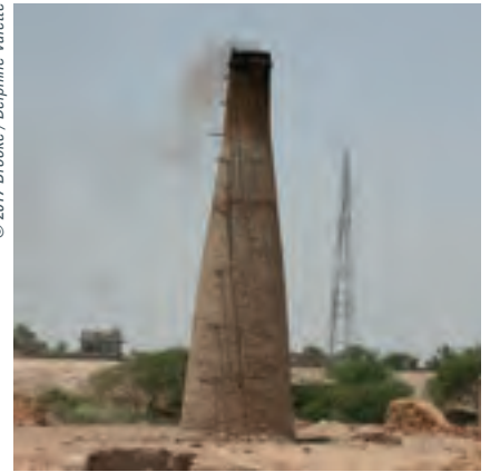
Fixed Chimney Bull's Trench Kiln
