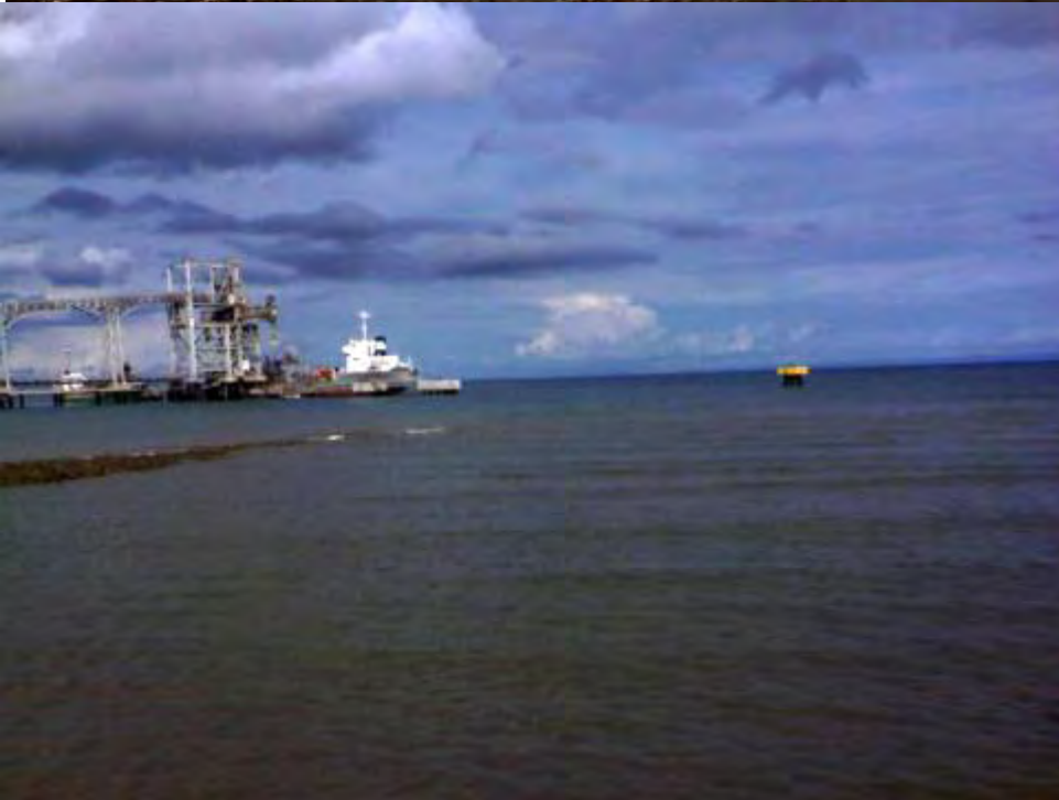
North Eastern Part of the Project Site
