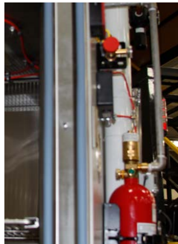
Fire Suppression Systems Inert Atmosphere Uses N 2 or CO 2 to eliminate Oxygen - does not prevent thermal runaway but can help contain
