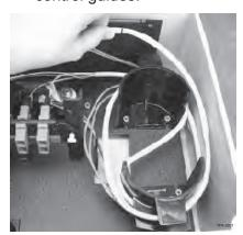
Step 2: Secure the tray to the wall as shown. Discard spacers depending on tray type..
