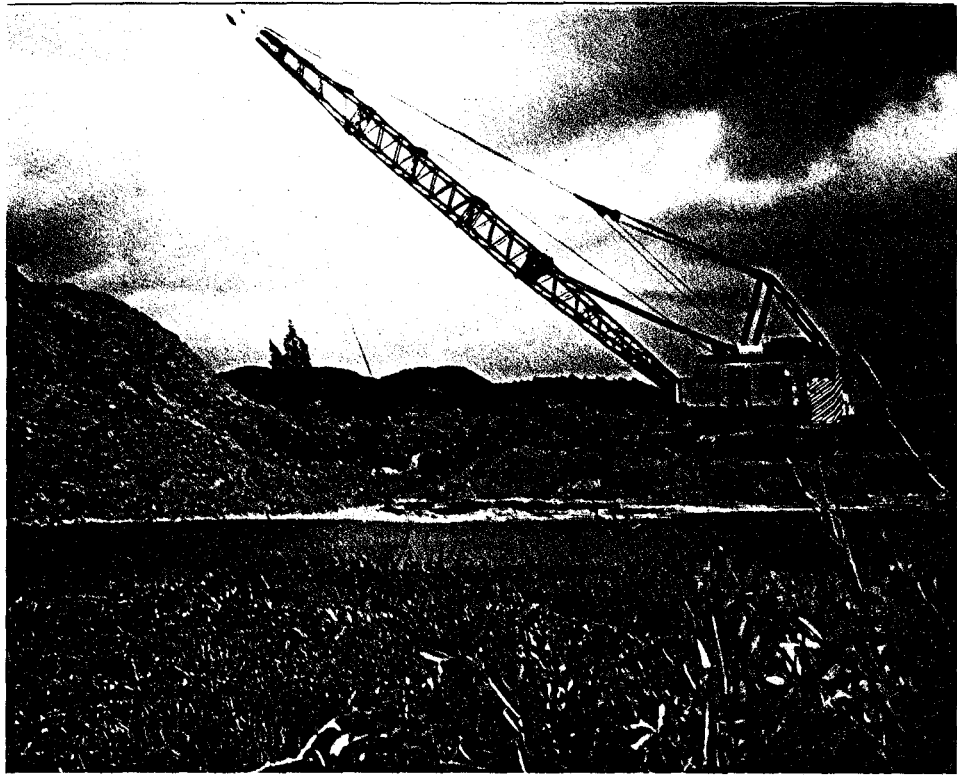
Photograph 3. Dragline building containment dike (Area 2, Fig. 4). Red and black mangroves of the area have already been destroyed.
