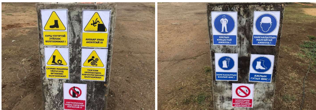
Photo 5: Warning Signs Placed at the Construction Site, Zuunkharaa TVET School
