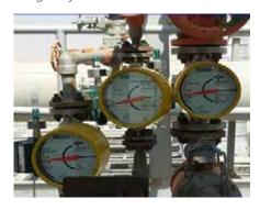
The implementation of wireless purge flow meters reduced gas emissions by cutting fuel gas consumption by 11%.
