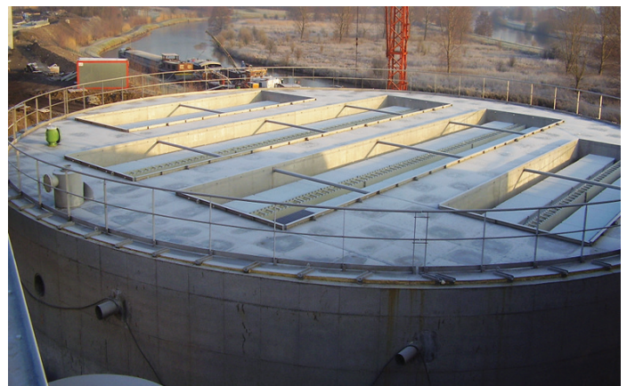
Claerebout, Belgium BIOTIM® UASB - 74,000 lbs COD/d - biogas: 353,300 ft 3 /d
