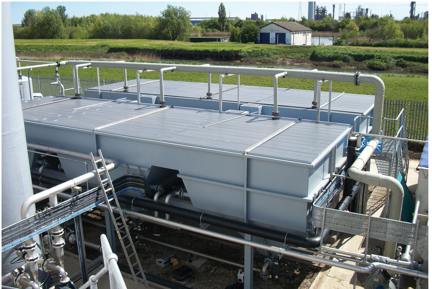
Mauri Hull, United Kingdom BIOTIM® UAC - Capacity: 74,250 lbs COD/day - biogas: 354,534 ft 3 /day
