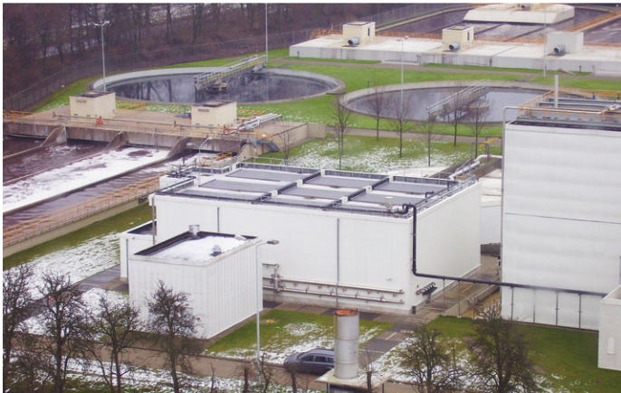
Heineken brewery, the Netherlands LUCAS® anaerobic - 30,000 lbs COD/d - biogas: 142,860 ft 3 /d
