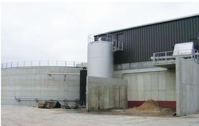
Agristo, The Netherlands BIOTIM® UASB - 64,000 lbs COD/d - methane: 305,600 ft 3 /d
