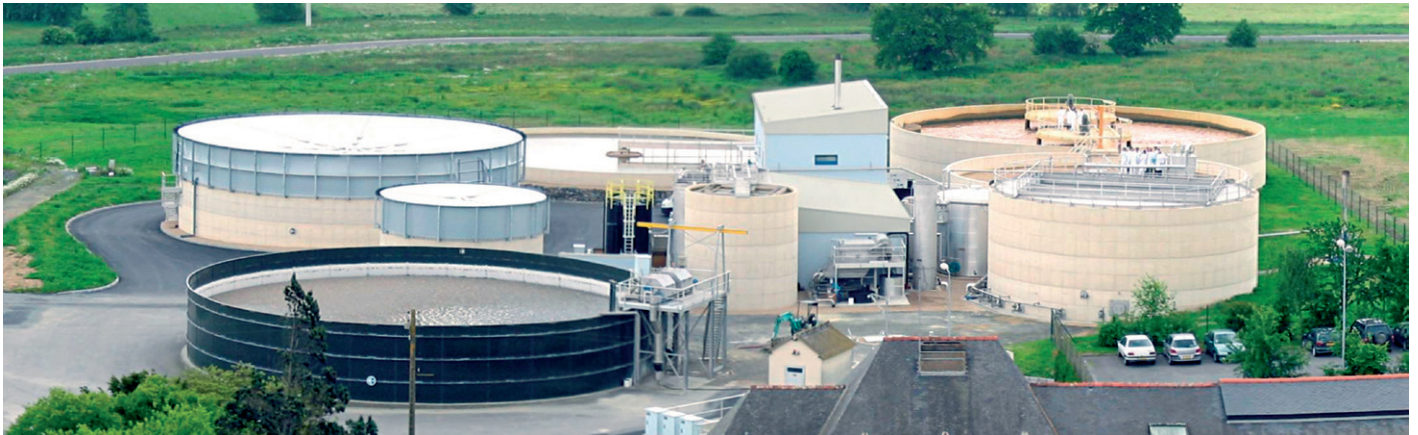
Lactalis Retiers, France - BIOTIM® UASB Capacity: 22,200 lbs COD/d - biogas: 105,050 ft³/d
