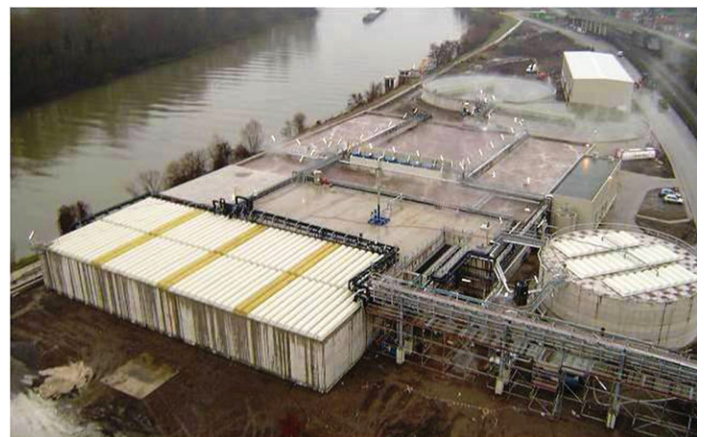
Biowanze, Belgium BIOTIM® UASB - 33,000 lbs COD/d - methane: 157,571 ft 3 /d
