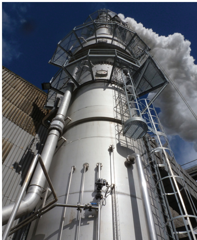
Tereos, France, dedusting + SO 2 and VOC treatment Wet dedusting and scrubber chimney Flue gas flow: 15,000.000 ft 3 /h
