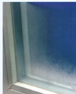
Full-Metal Spacer With conventional metal spacers, condensation is a fact of life.
