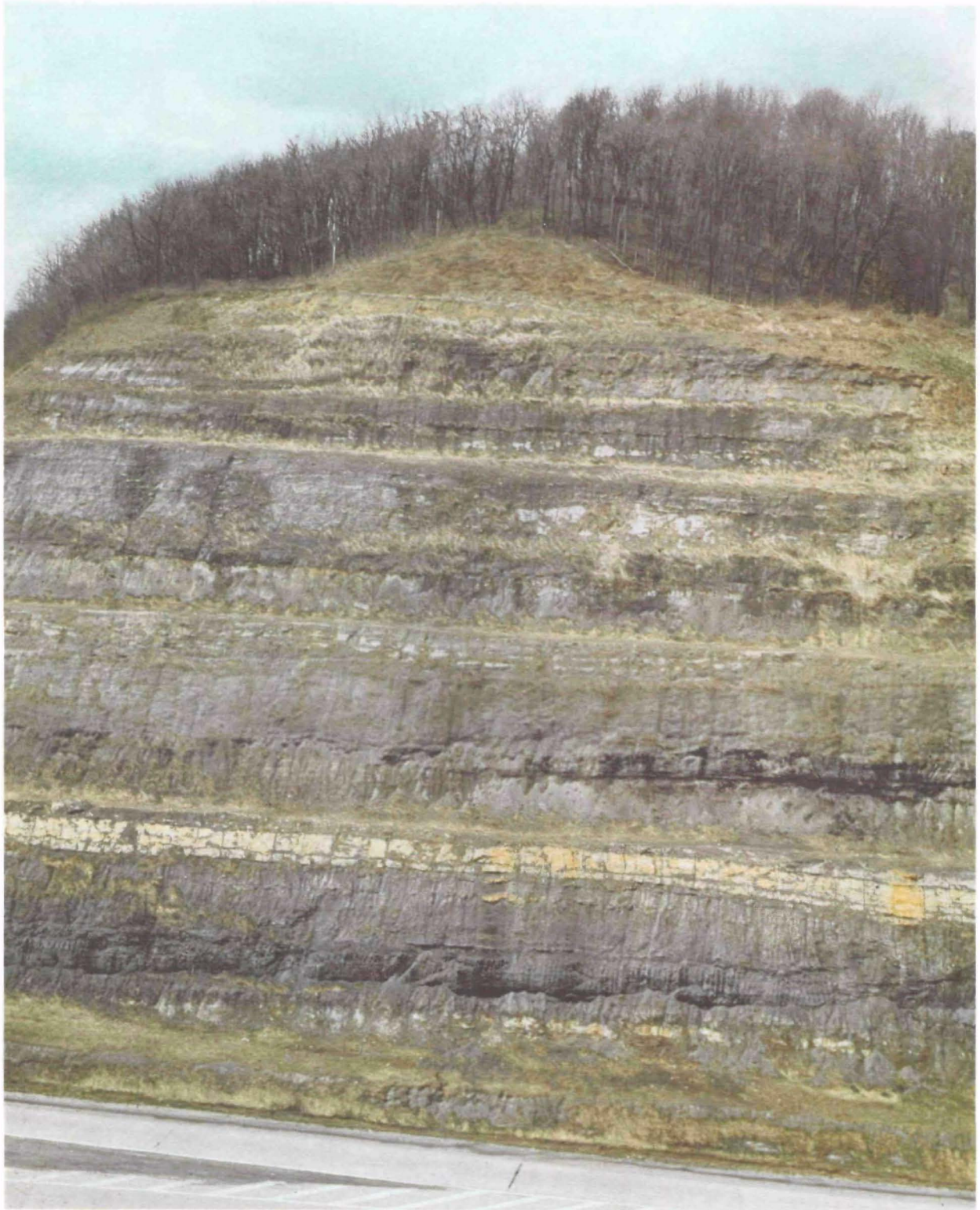
Figure 3. Pittsburgh-Redstone overburden showing yellowboy staining on the limestone between the coal seams.
