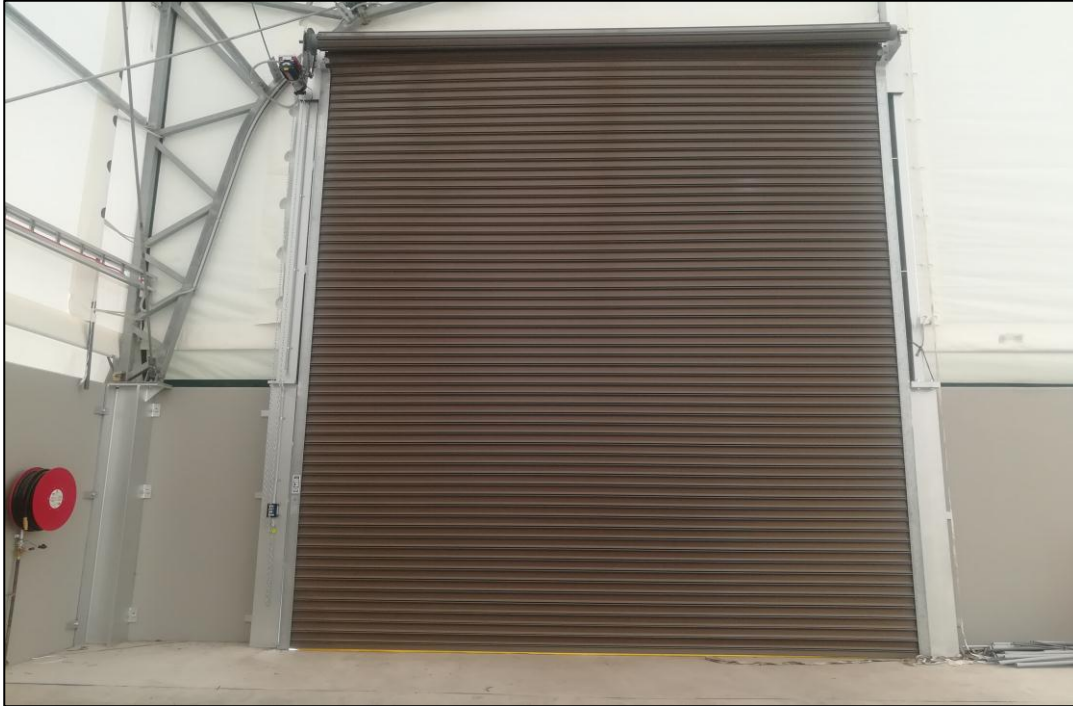
Figure 12 - Roller Doors-Yatala QLD. Invessel Compost Facility
