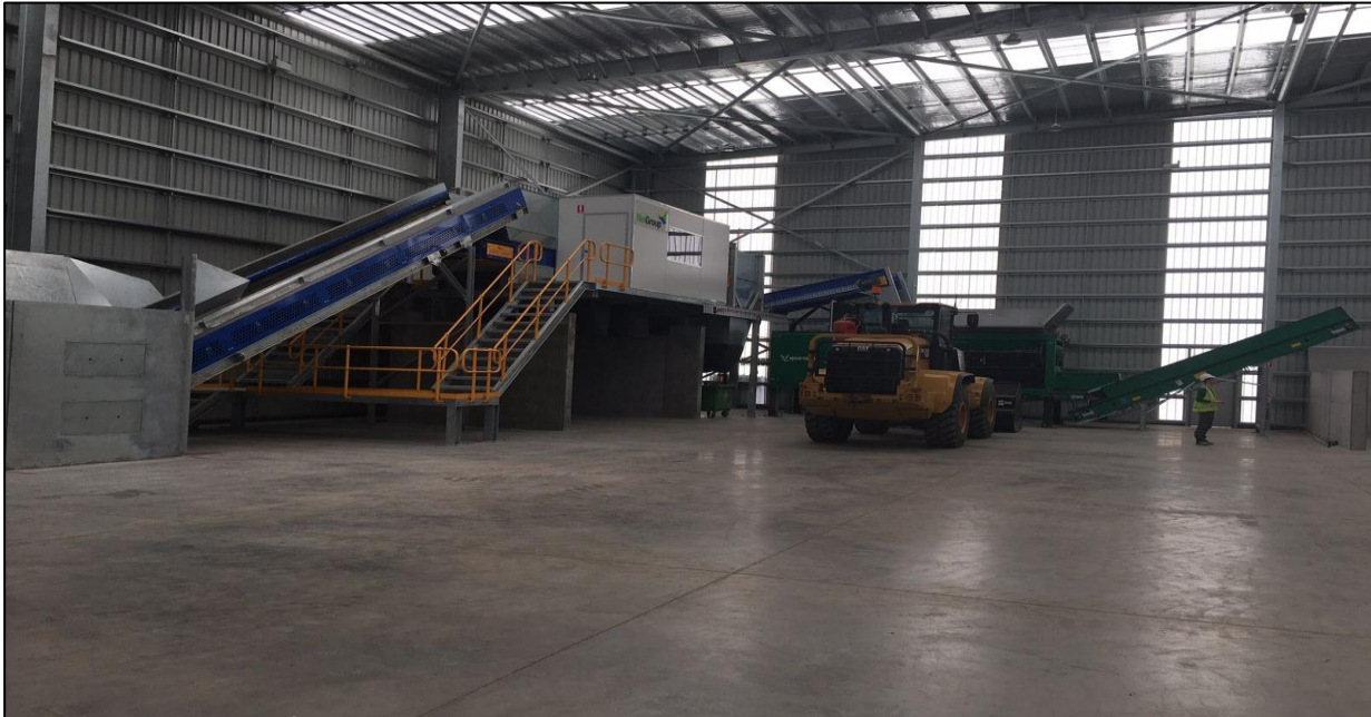
Figure 15 - Decontamination Area - Shell Harbour NSW Invesel Compost Facility
