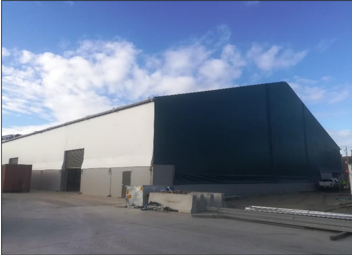
Figure 11 - Receival Building- Shell Harbour NSW Invessel Compost Facility
