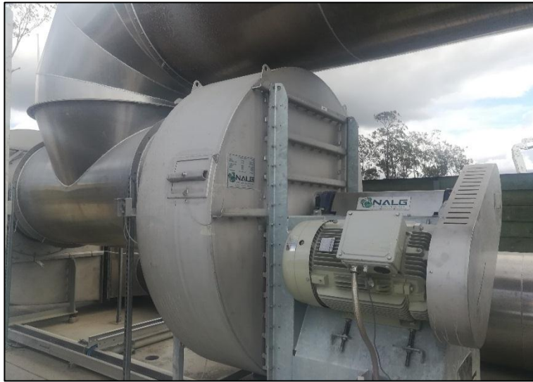
Figure 30 - Bio-filter blower
