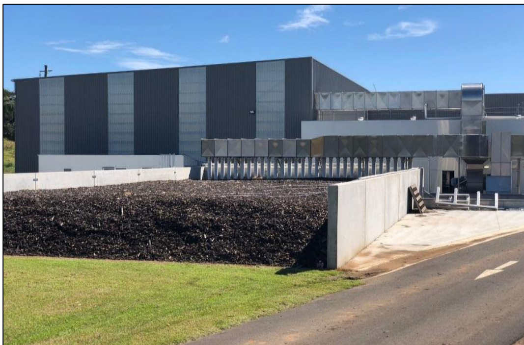
Figure 26 - Bio-filter - Shell Harbour NSW Invesel Compost Facility
