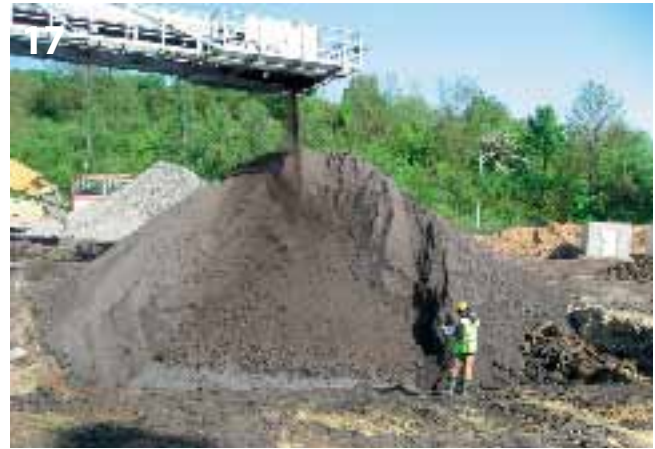
An initially good result of the “dry” muck production attempt, which failed after 75 m with the ingress of the groundwater and generation of sticky muck
