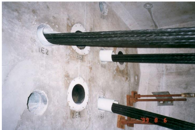
Example of installation of PE sheathed FLOGARD™
