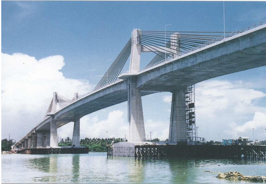
The second Mactan Bridge (Philippines) : ECS stay cable
