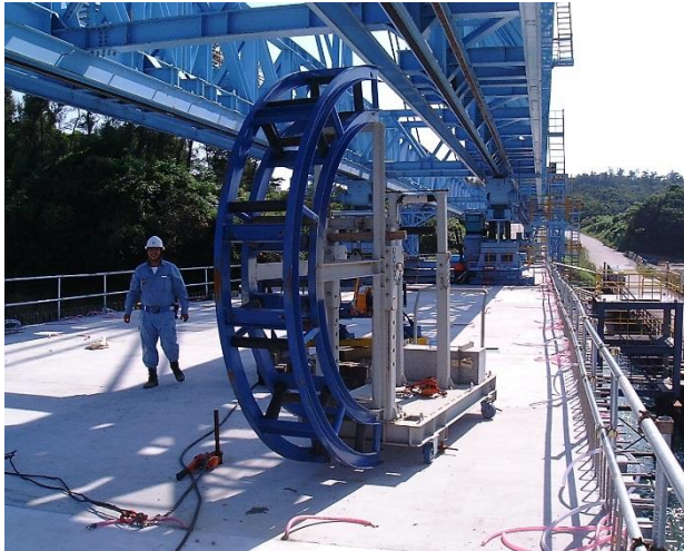
Specially designed turn roller for ECS
