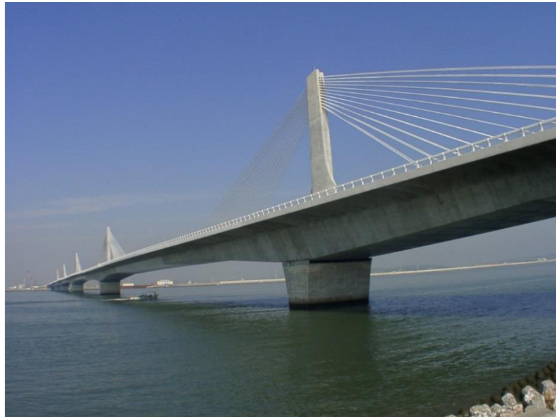
Japan Highway Corp. Ibi-gawa bridge (2002)
