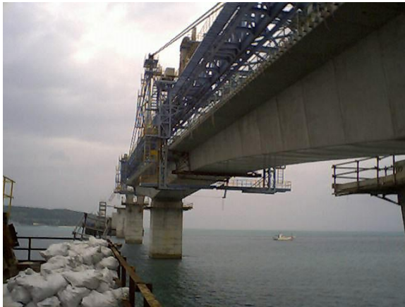
Kouri Bridge ( Okinawa., Japan)
