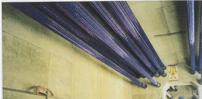
Installed ECS as external tendon inside of girder (Ibi Bridge : FLOGARD™)
