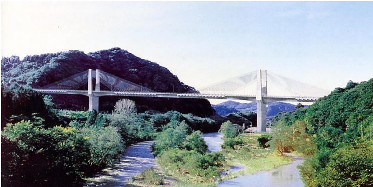
Samonoe-Bokyo-Onashi Bridge ( Aomori, Japan ) :
