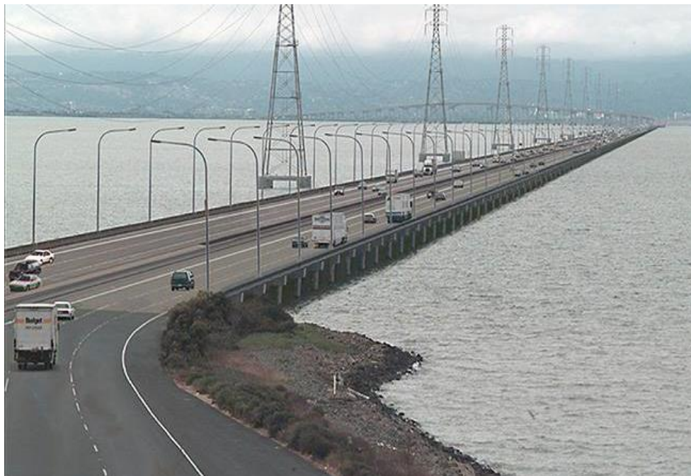
San Mateo Bridge (California, USA)
