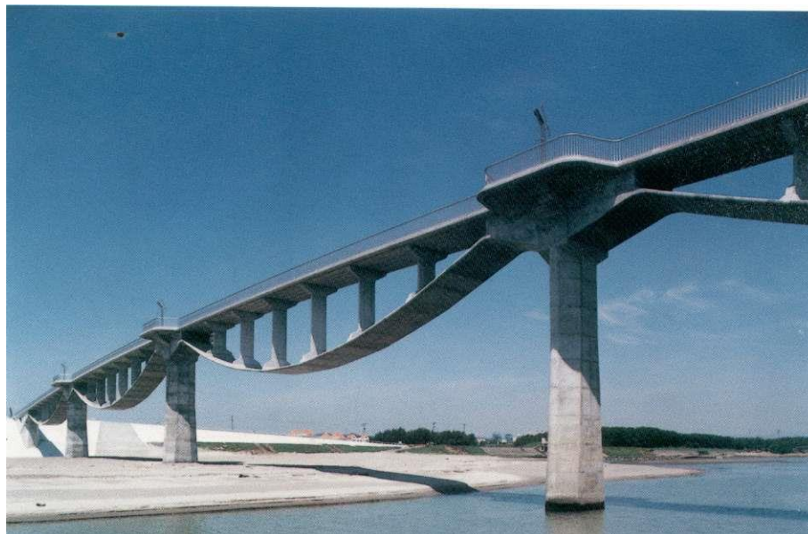
Shiosai Bridge (Shizuoka, Japan) : applying ECS, FLOBOND™, for inner cable
