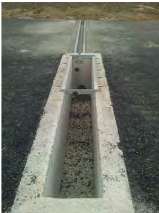
Concrete Case for water obstacle
