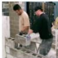
Workers use the two-man lift technique to reduce stress of lifting and twisting.
