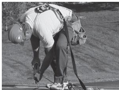
Construction work: fastening down roofing material
