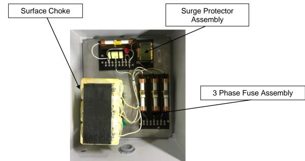
Figure 24: Surface Choke and Surge Protector Assembly 90B2175
