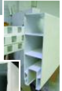
Interior construction of 7" rail
