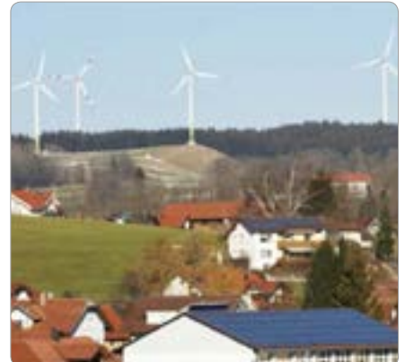
The research Rumph does helps governments, energy suppliers, energy services providers and grid operators in the development of products, services and related regulation (Photo: Siemens)
