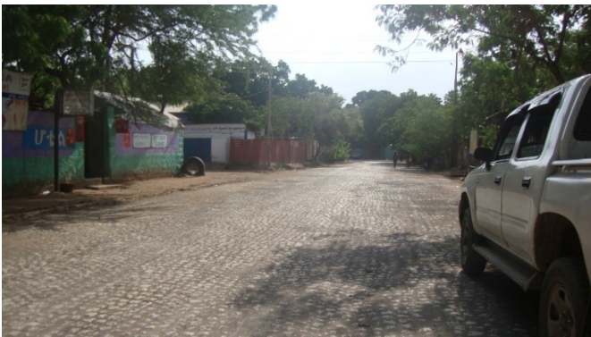
Source: PPT Cobblestone Development under Urban Local Government Development Project. Note: June 2013.
