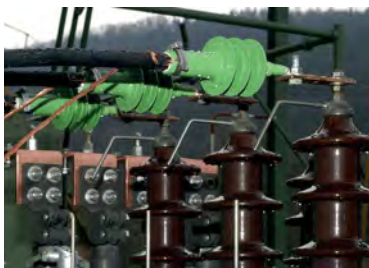
AFN10 as a transformer connection
