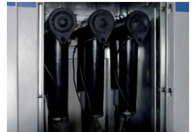
SF-6 system connection with 480TB+800SA
