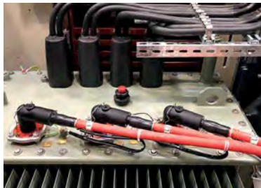
Transformer connection with 200LR
