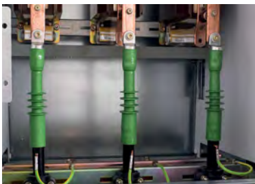
AIS20 with mechanical cable lug
