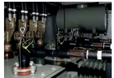
Transformer connection with 158LR
