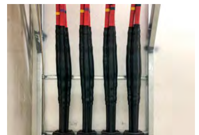
24CSJA-S cold-shrinkable straight joint
