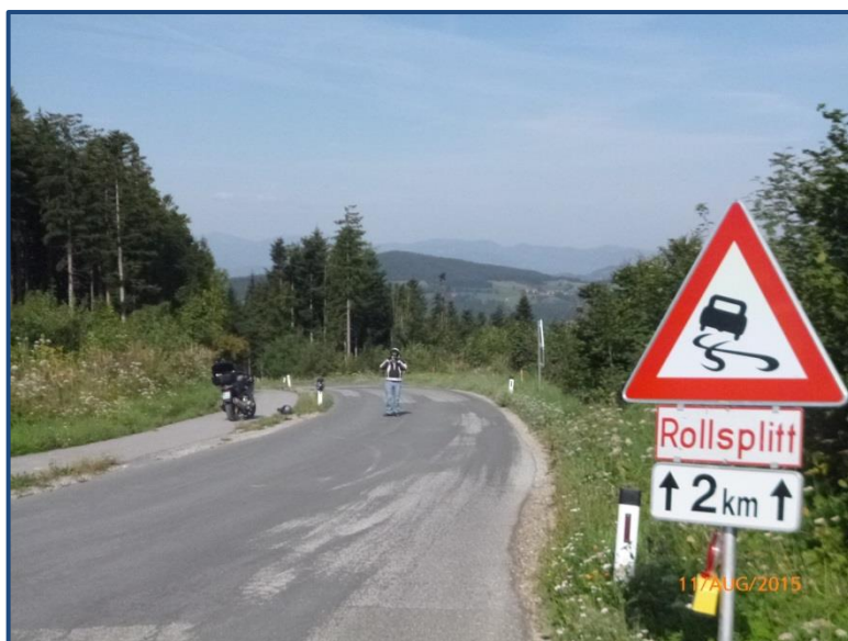
P1140667: Loose gravel at the 4-way intersection. The sign is only visible to straight through traffic!
