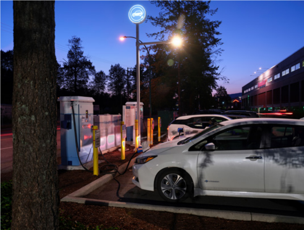
Figure 5: Example of a BC Hydro light pole assembly
