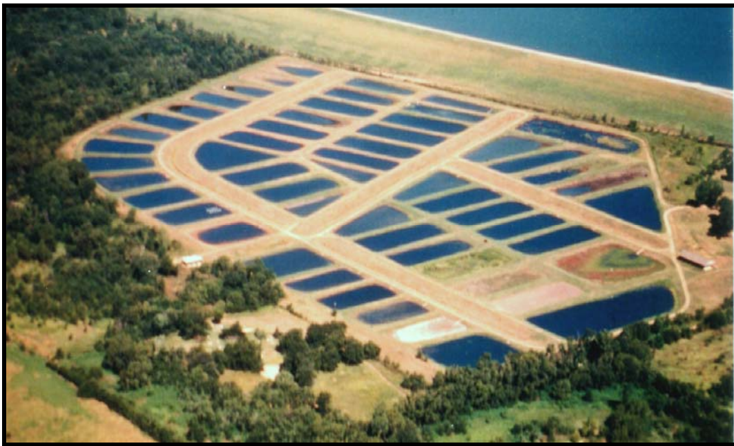
Figure 7. Aerial view of the Lewisville Aquatic Ecosystem Research Facility – Lewisville, Texas.
