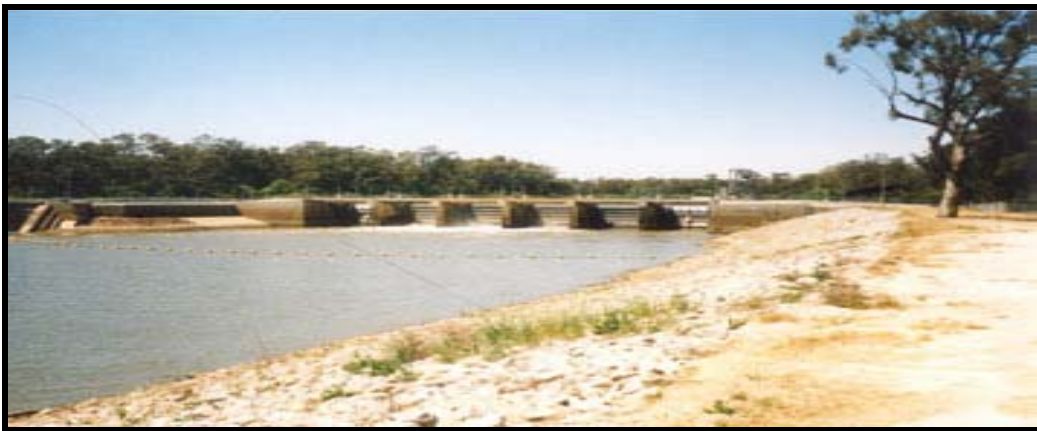
Figure 5. Murray River, Australia common carp barrier; Photo credit: Environmental Waikato.
