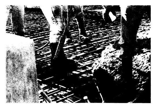
Fig. 3.28: Vibrating of Fresh Concrete at North Main Street Eastbound
