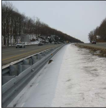
Figure 9. Modified Thrie Beam Median Barrier – New Jersey Route 80, Morris County
