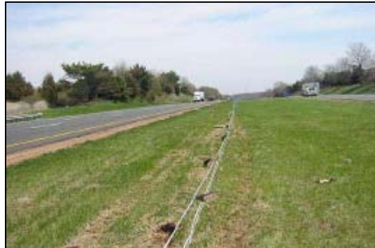
Figure 37. Impact 8: Barrier Damage
