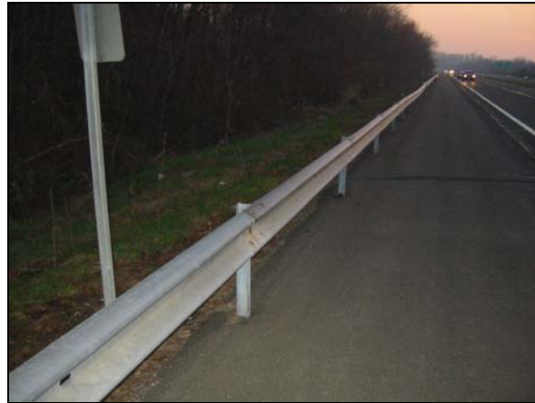
Figure 8. Weak Post W-Beam Roadside Barrier – Southbound New York Thruway
