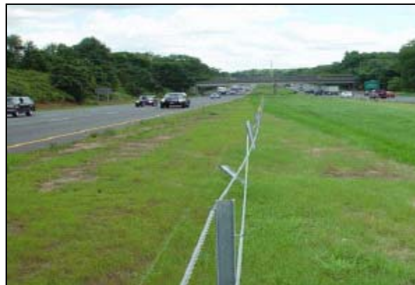
Figure 38. Impact 9. Barrier Damage
