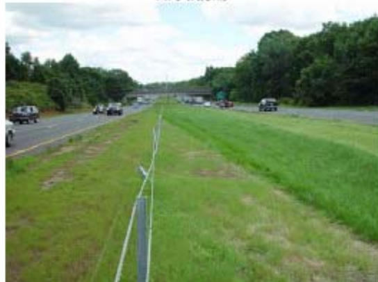
View Approaching Site
