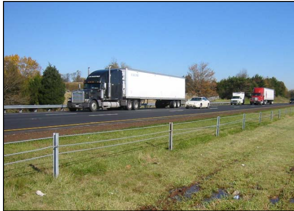
Figure 3. Three Strand Cable Barrier – New Jersey Route 78, Hunterdon County
