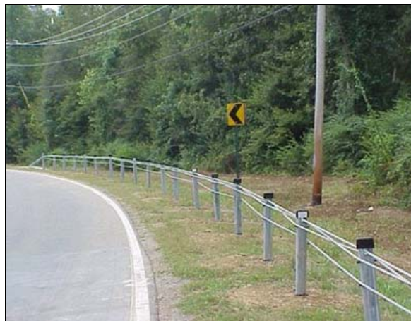
Figure 6. Brifen Wire Rope Safety Fence – US Version (14)
