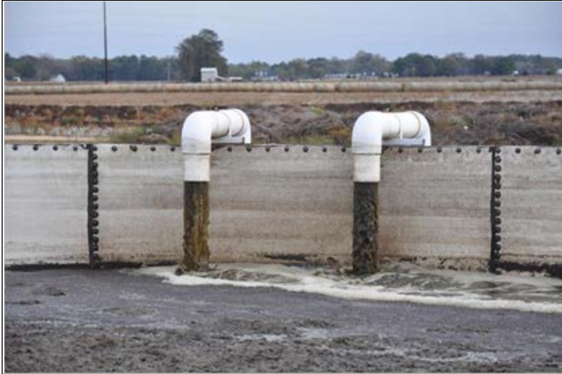
Raw manure from the finishing farm being transferred into the homogenization tank.
