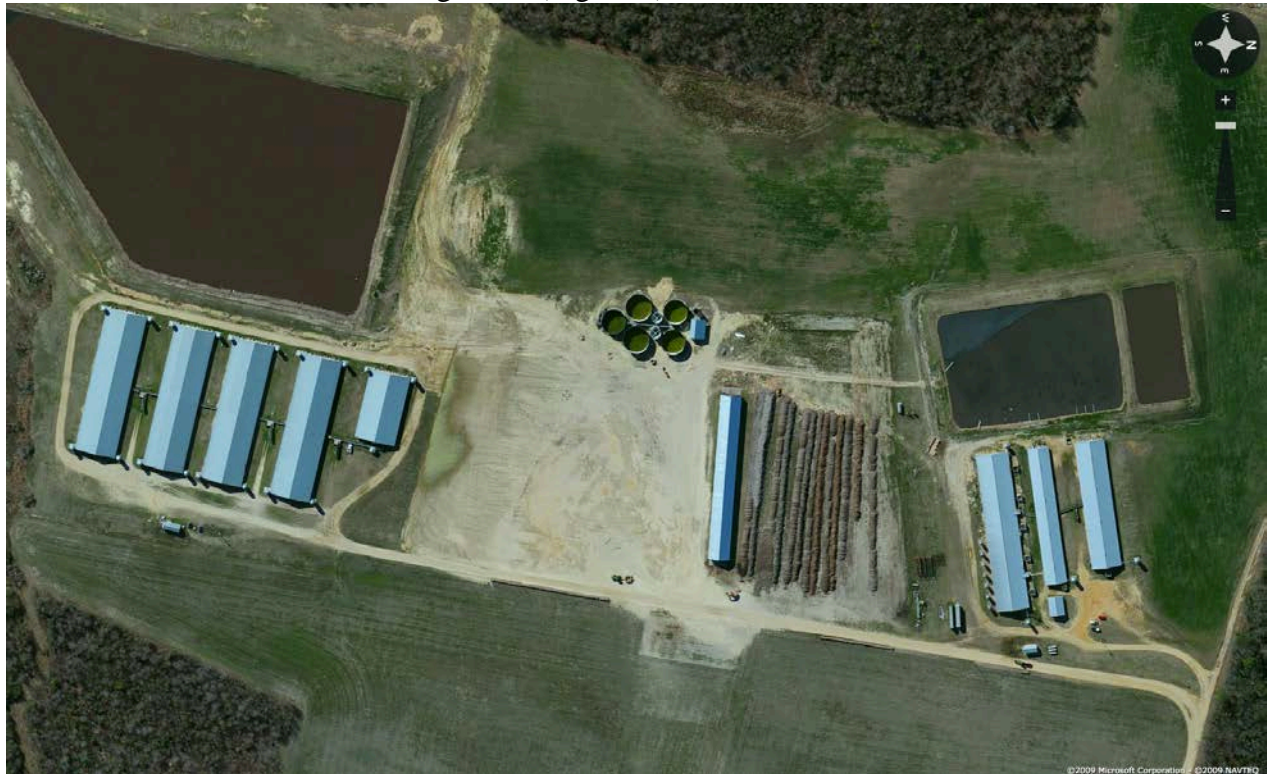
Figure 3. Terra Blue Gen 3 wastewater treatment system (tanks in center) that replaced the lagoon treatment at Jernigan farm. The system provided treatment to all the manure from a 1200-sow (farrow to feeder) farm (three barns shown at right) with flushing system, and a 12,960-head feeder to finish farm (four and a half “quad” barns shown at left) with pit-recharge system. Photo source: Flashearh.com.
