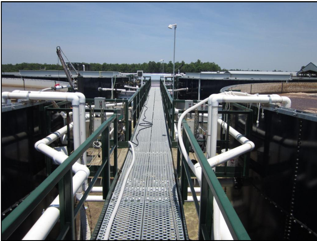
View of treatment plant from the catwalk.
