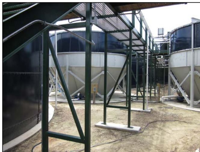
Picture shows view of plant at ground level. Cone bottom tanks are settling tanks used in nitrogen (left) and phosphorus (right) modules.
