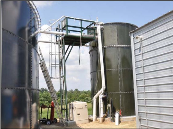
Homogenization tank receiving raw manure flush from finishers (left) and decanting tank sludge (right). In the upper left is the ultrasonic probe that monitored liquid levels.
