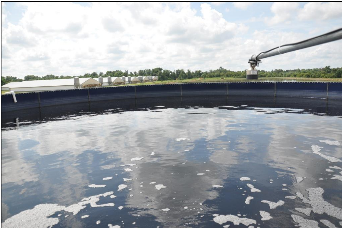
Clean water tank. It stored N treated water for recycling into the barns.
