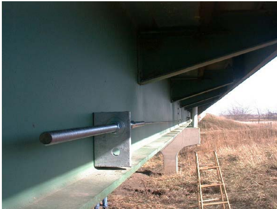
(b) Top CFRP bar in place
