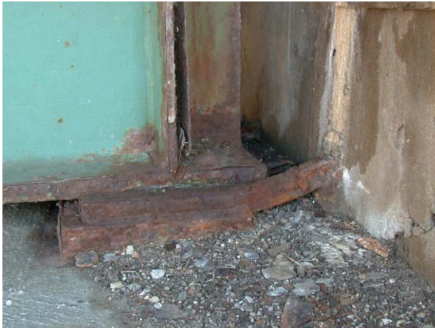
(d) Typical east abutment condition
