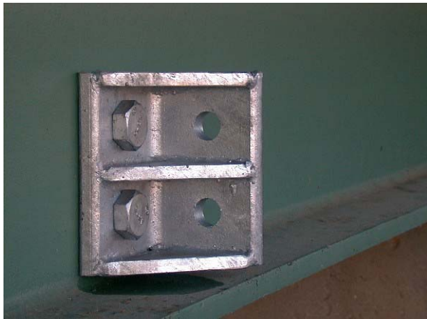
(a) Stiffened steel angle assembly
