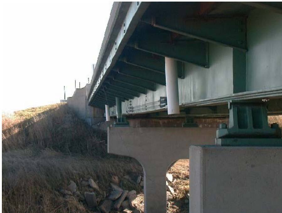
(c) CFRP bars in center span
