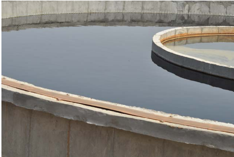
Figure 12: Clariflocculator
