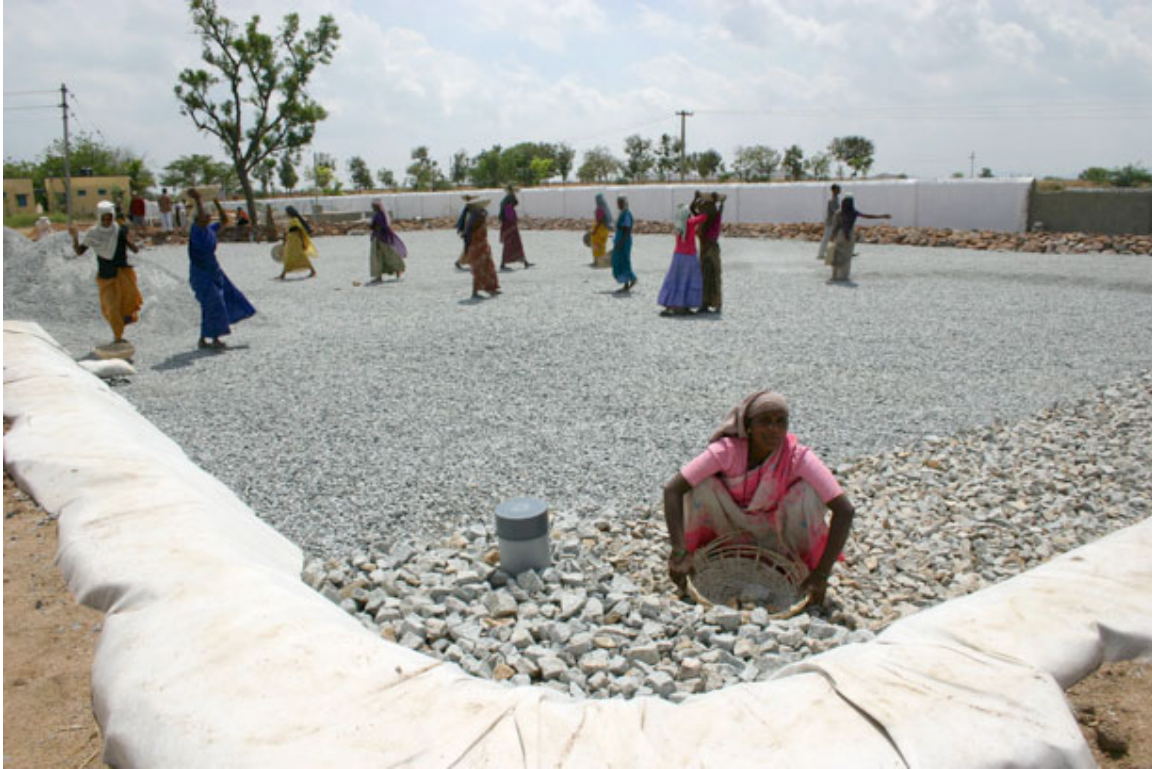
Figure 18: Filling the site with gravel and water distribution piping
