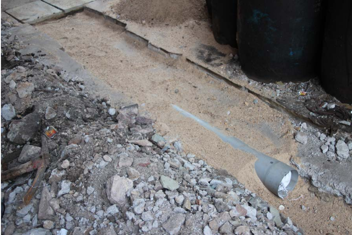
Figure 15: Recycled water pipeline being constructed at Kothari Textile Facility
