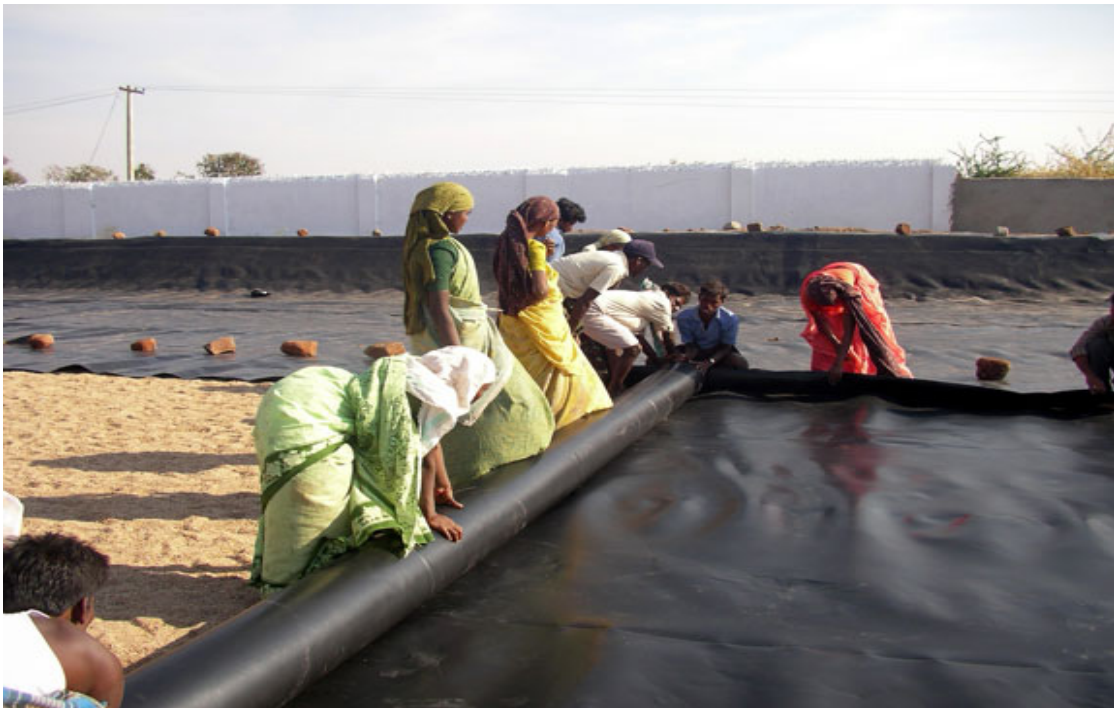
Figure 17: Laying a liner in the soon to be wetland bed
