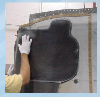
Smoothing kit into sanded recess, tool located and template aligned
