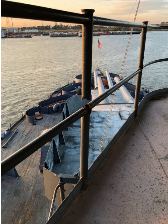
Figure 20 - Representative handrail rust damage needing repair.
