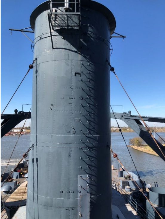
Figure 16 - General photo of the smokestack
