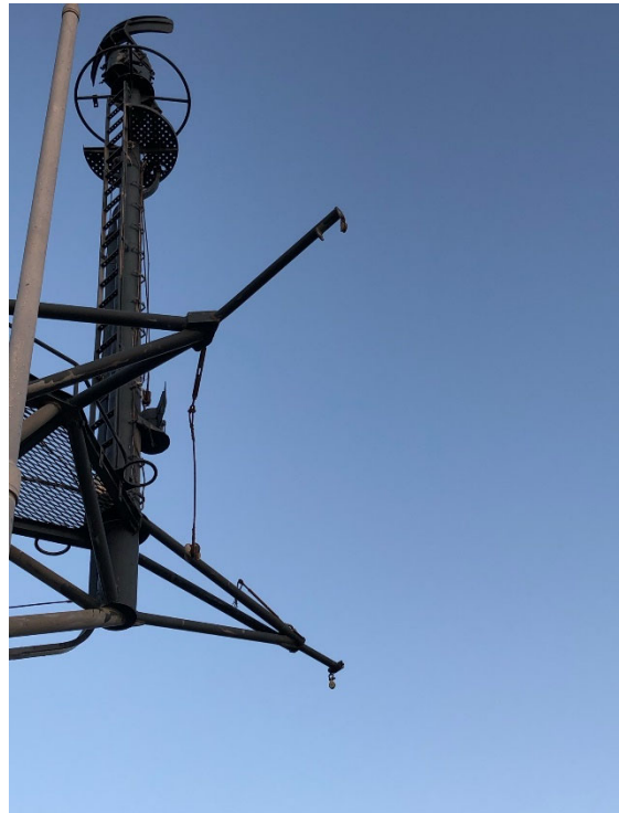
Figure 23 - Broken stays for radar topmast needing replacement.
