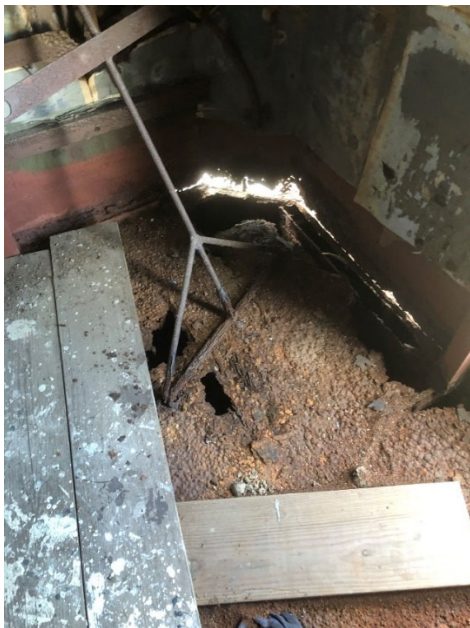
Figure 12 - Rusted out lower bulkhead and deck of Sky Control Forward in foremast.
